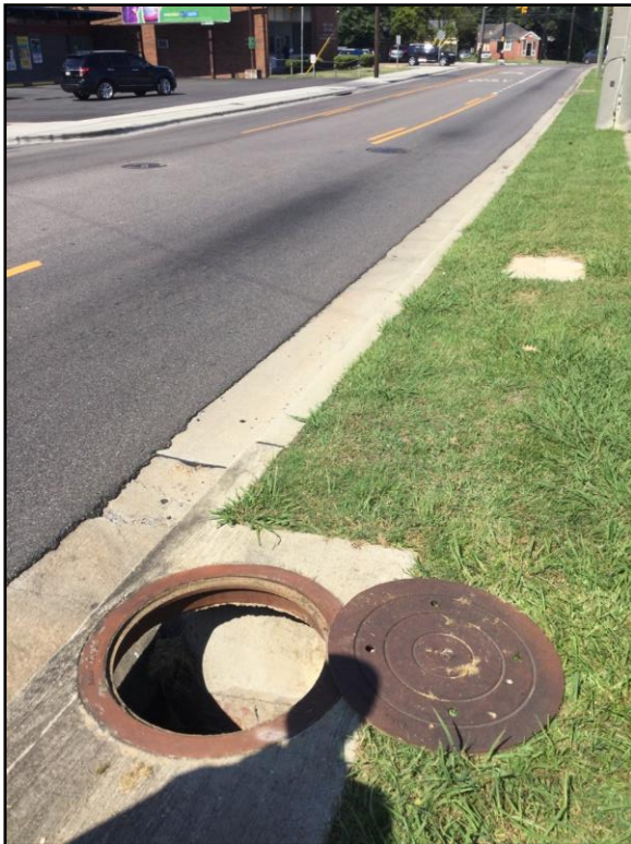
Photo 10: View of outfall 9 out.
