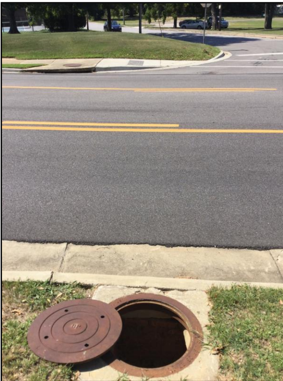
Photo 14: View of outfall 11 out.
