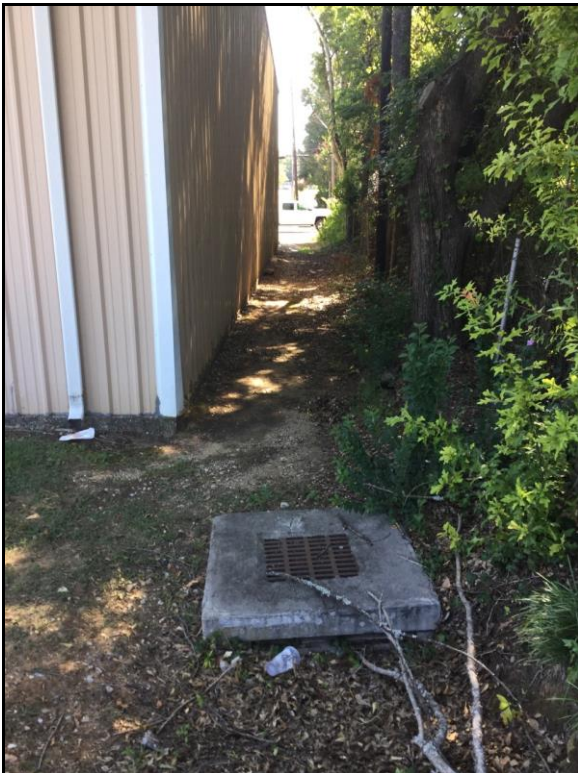
Photo 2: View of outfall 5 out.
