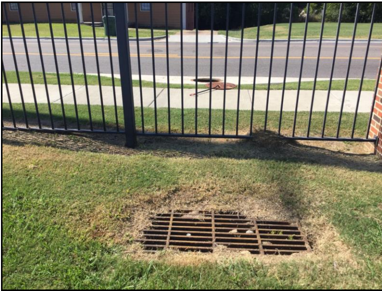
Photo 6: View of outfall 7 out.
