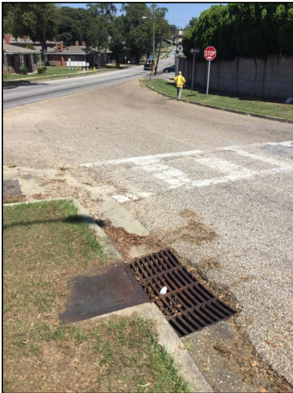
Photo 18: View of outfall 13 out.
