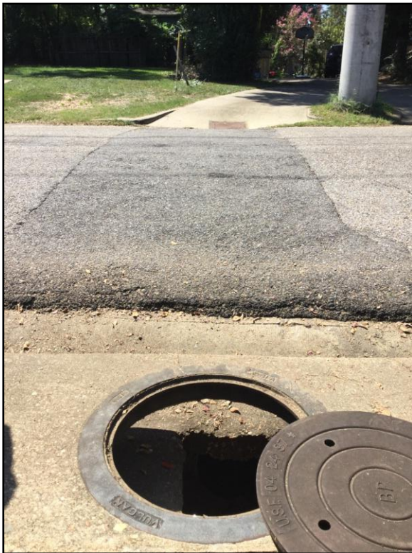
Photo 16: View of outfall 12 out.
