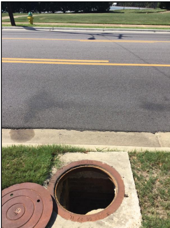
Photo 12: View of outfall 10 out.
