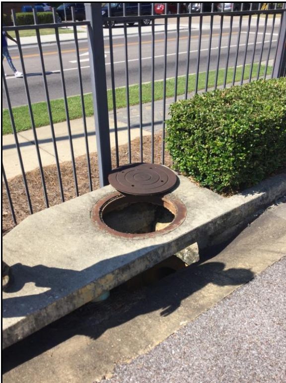
Photo 8: View of outfall 8 out.
