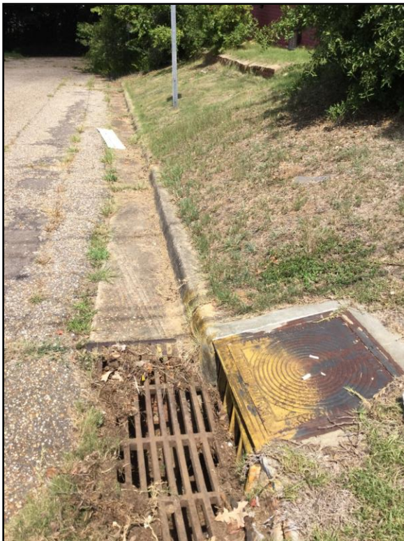
Photo 26: View of outfall 17 out.
