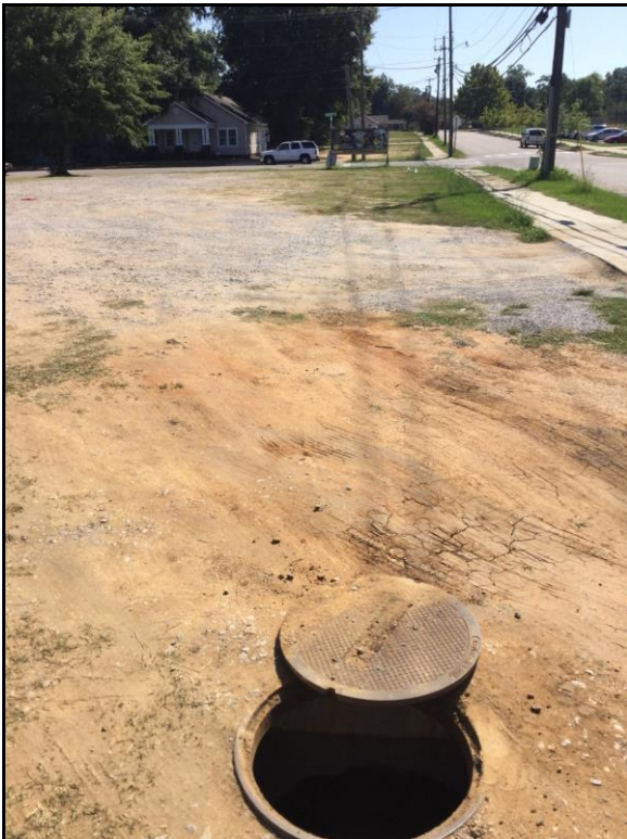
Photo 4: View of outfall 6 out.
