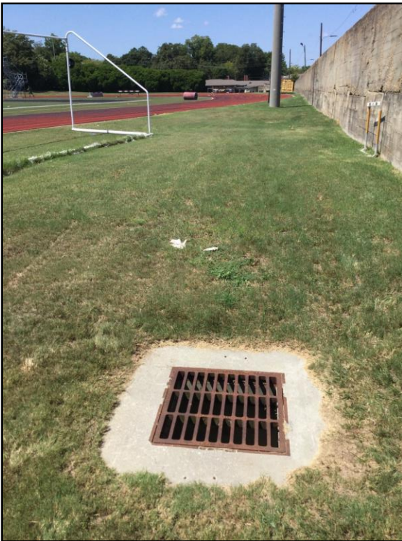
Photo 22: View of outfall 15 out.
