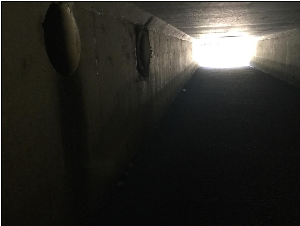
Photo 24: View of outfall 16 out.
