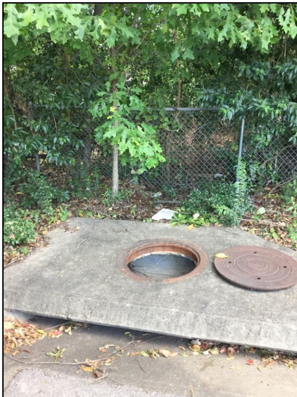
Photo 28: View of outfall 18 out.
